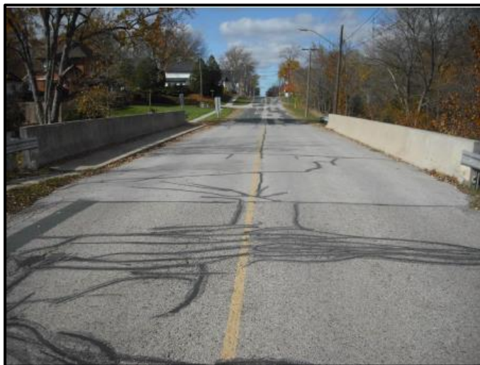
Main Street Bridge (BCI = 98.8 Very Good)
